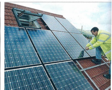
POWER OF THE SUN: Solar panels being installed
